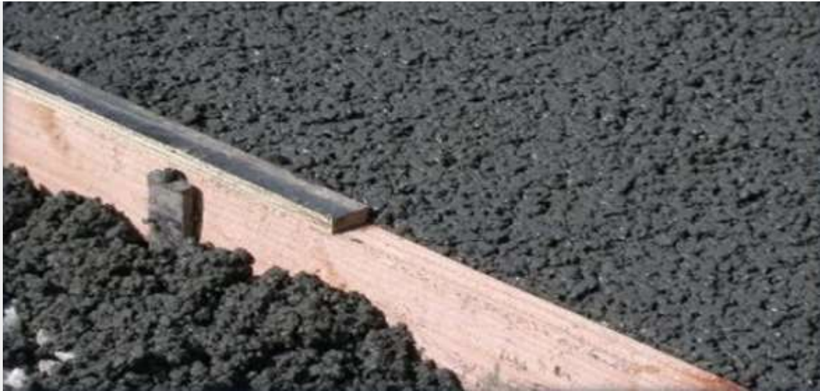
Fig-7 No Fines Concrete
