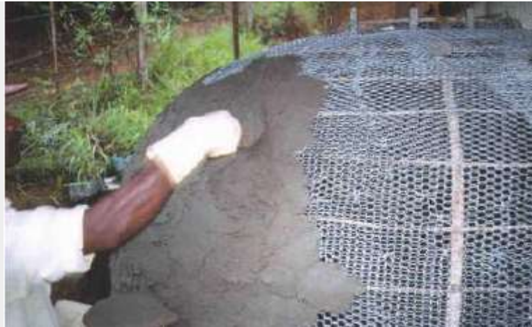
Fig-14 ferro concrete
