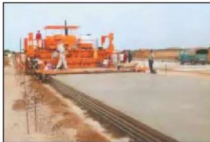
Fig-6 placing of concrete
